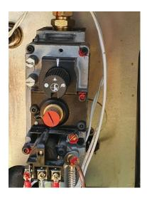
2. Locate pilot light hole. Use long reach lighter through the pilot hole to ignite the pilot light. Alternatively, if no long-reach lighter is available light from underneath. This step may take a minute or two.
